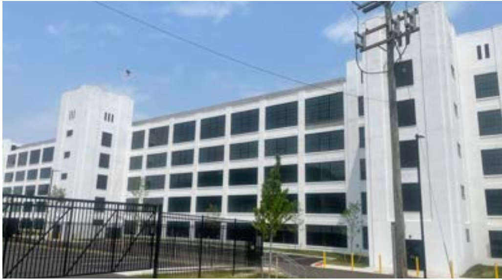
EJ Victory Building Rehabilitation
